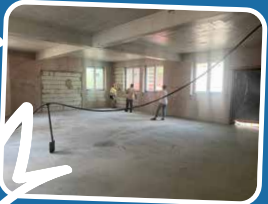
JULY 22 THE ROOM AFTER REMOVING ALL TILES, DEBRIS, ETC.
