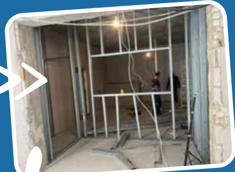
SEP22 ANOTHER PLACING CONSTRUCTION JOB INVOLVES THE PROFILES FOR THE WALLS
